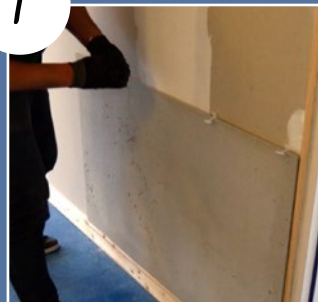
POSITION THE WEDGES AT REGULAR SPACES
