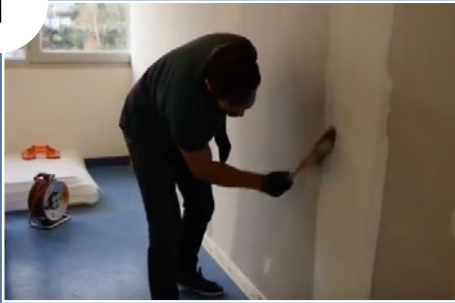
CLEAN THE AREA BEFORE THE INSTALLATION
