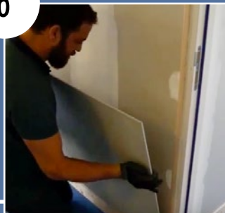
PLACE THE PANEL STARTING WITH THE BOTTOM
