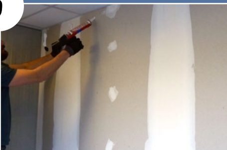
APPLY GLUE ON THE WALL (OR ON THE PANEL)
